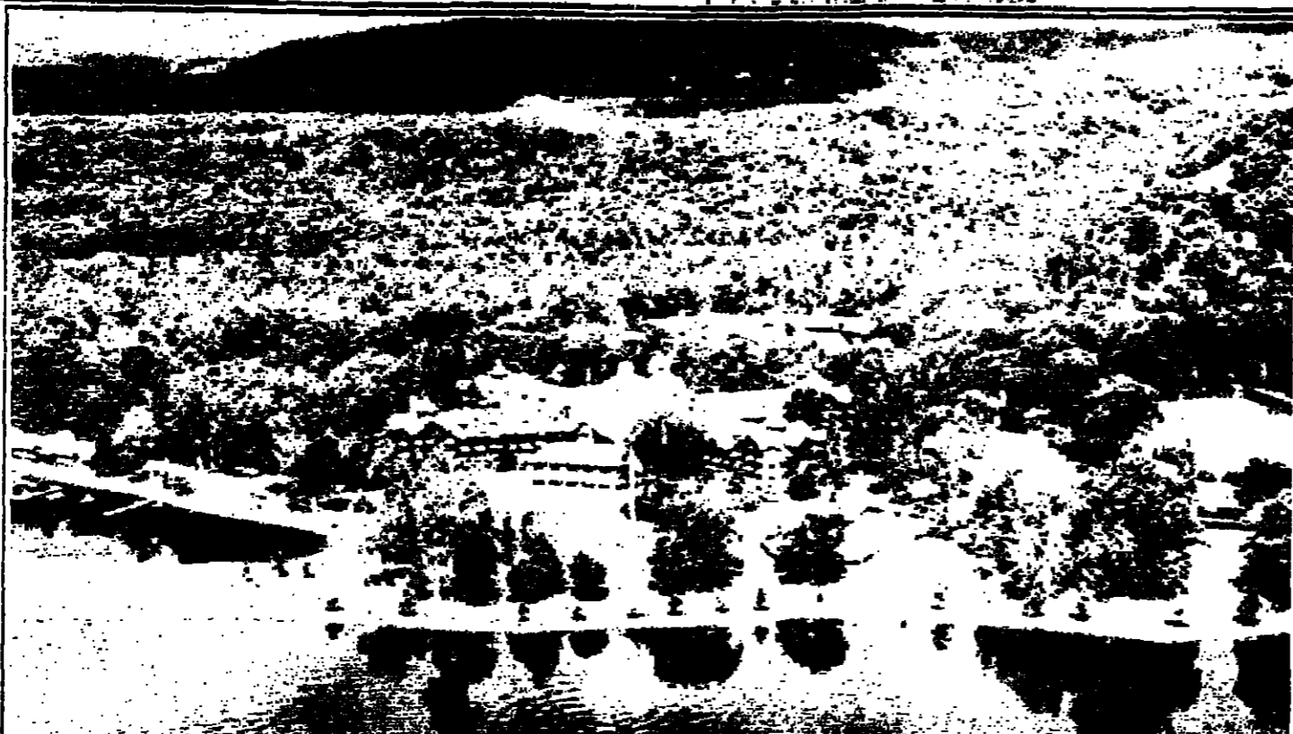
SUMMIT LODGE: The luxurious Chateau Montebelle will be the home for the leaders of the United States, Britain, France, West Germany, Japan, and Italy when they attend the economic summit in Ottawa next week. The chateau is the biggest log structure in the world and was built in three months in 1939. Montebelle is located 40 miles east of Ottawa.
